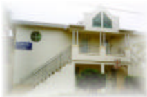
Community Court building
